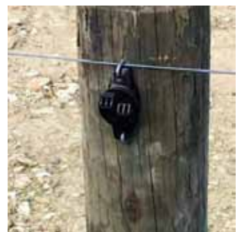
Below: re-work is waste – farm worker thought he was doing what he was told when asked to fix the electric fence to the posts – just didn't think to put the wire through the insulators . . .
